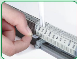
Installing adjacent jumper
