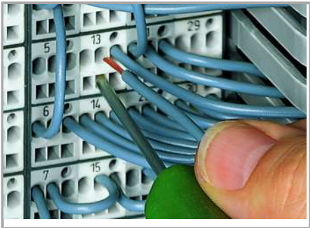
CAGE CLAMP® connection
